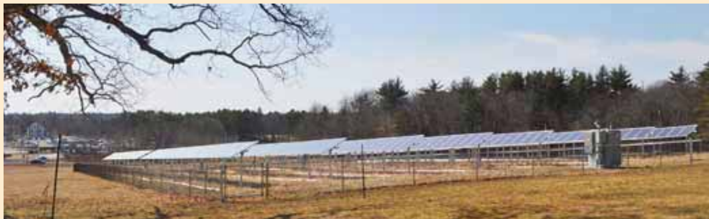
Both crops and solar power compete for the sun's energy at the Northeastern Correctional Center in West Concord. This solar array was sited on good quality farmland that had excellent southern exposure.
